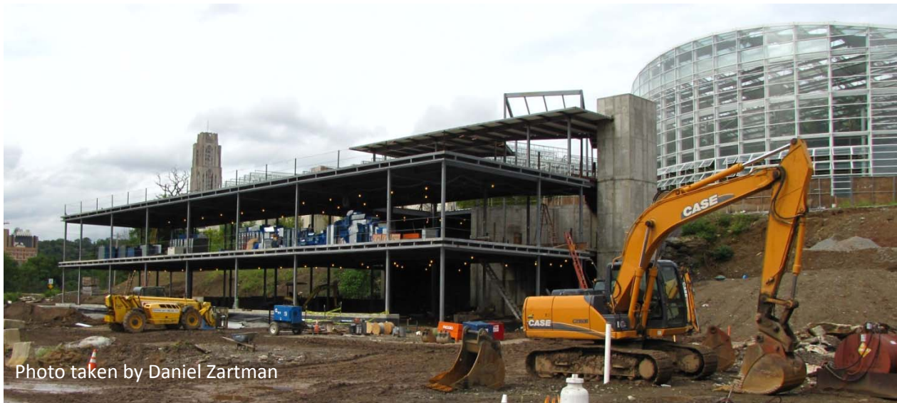
Figure 3 - Concrete and steel superstructure taken September 7, 2011.
